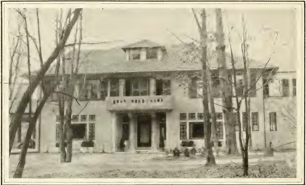
FIG. 4. A CONCRETE HOUSE, COMPLETED.
